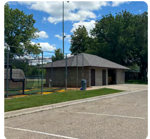
Main storage building in the park
