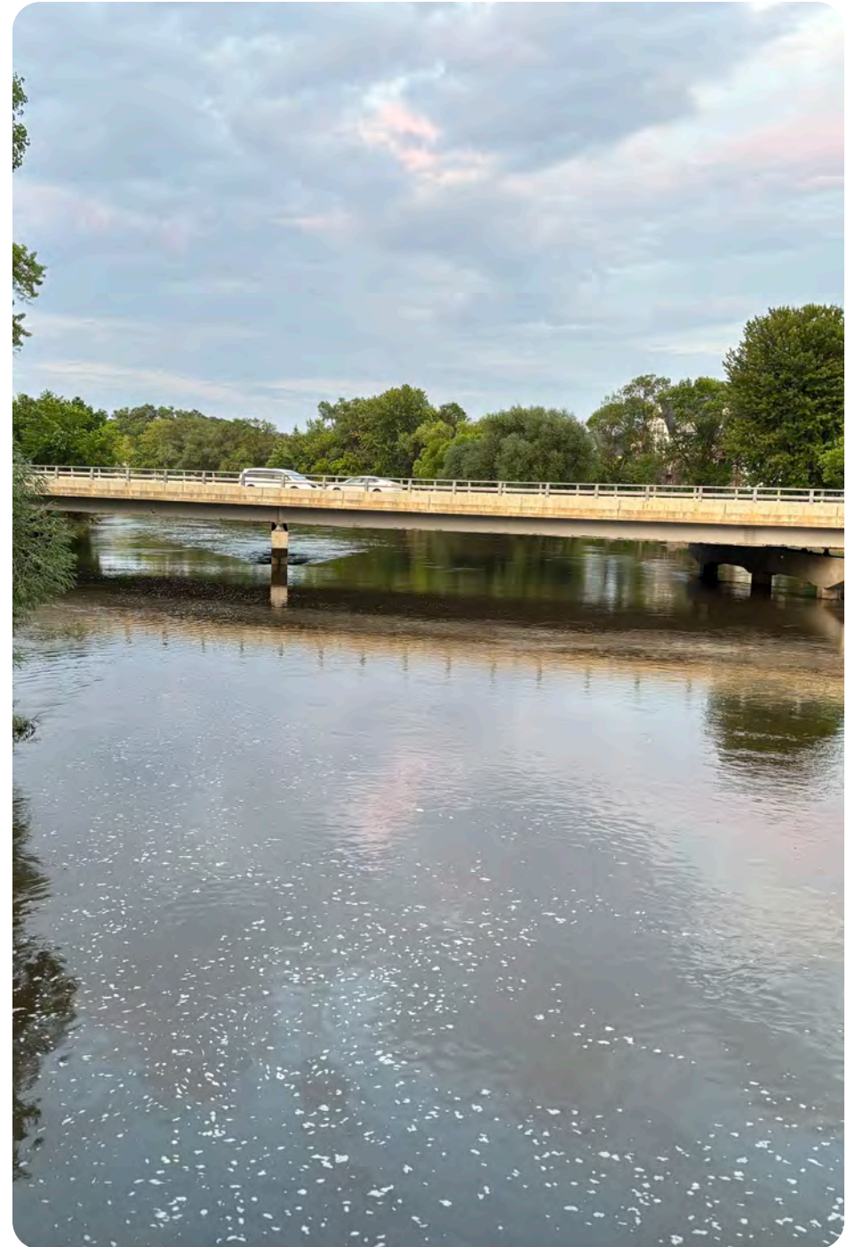
View of MN-3 from the pedestrian bridge
