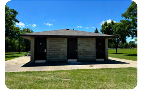
Picnic shelter's indoor restrooms
