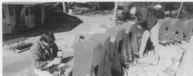
17. Glen Echo Park near Washington, D.C., is an early 20th century amusement park. (It is the home of the first bumper car ride in the world.) Its neon signs needed repair: (a) tubes were broken and the surrounding "metal cans" needed work also; (b) and (c) removal of the back of "Candy Corner" sign revealed debris from insects and birds; (d) preparing the "metal cans" from the "Pop Corn" sign for remounting; (e) and (f) neon fabricators installing the new tubing in the repaired and remounted cans; (g) repairs finished, the relit signs enliven the park once again. Photos: (a-c) Stan Fowler; (d-f) Larry Kanter; (g) Rebecca Hammel.
