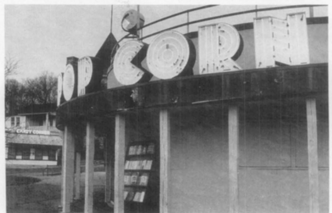
17. Glen Echo Park near Washington, D.C., is an early 20th century amusement park. (It is the home of the first bumper car ride in the world.) Its neon signs needed repair: (a) tubes were broken and the surrounding "metal cans" needed work also; (b) and (c) removal of the back of "Candy Corner" sign revealed debris from insects and birds; (d) preparing the "metal cans" from the "Pop Corn" sign for remounting; (e) and (f) neon fabricators installing the new tubing in the repaired and remounted cans; (g) repairs finished, the relit signs enliven the park once again. Photos: (a-c) Stan Fowler; (d-f) Larry Kanter; (g) Rebecca Hammel.
