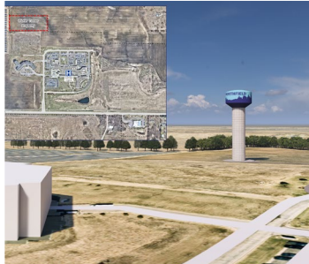
NW area water tower
