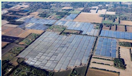
North Star Solar 100-MW project
