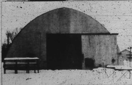
HACKENSACK QUONSET BECOMES STUDIO
