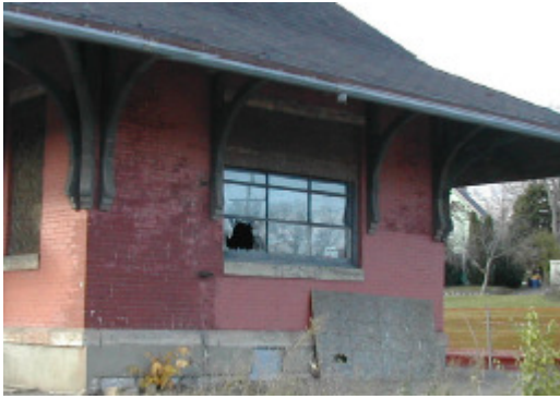
Large window on the north end of the depot.
